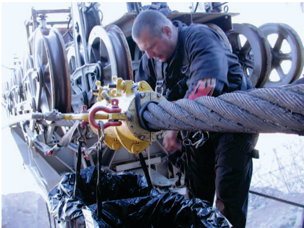
Hoover Dam Trolley before lubrication 3-12 inch (89mm).
